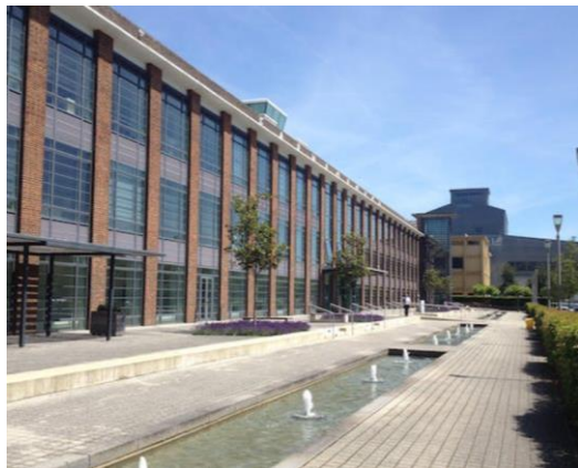
Figure 6 Image of The Hub
